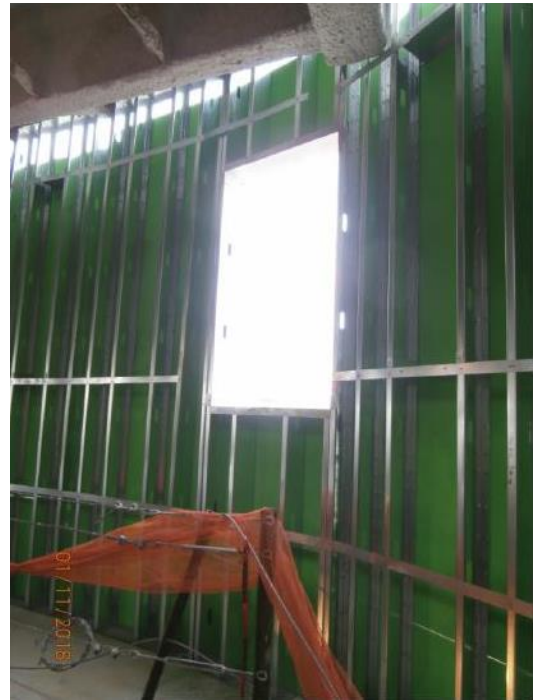
Interior - Curved punched opening to support eccentric window system
