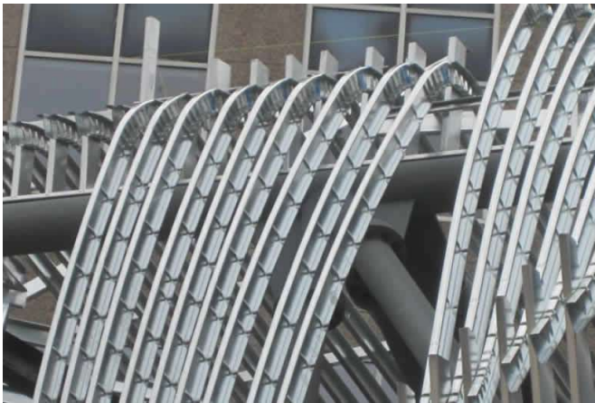
Exterior Picture of Curved/Radius Studs Bent to Different Radius. Photo courtesy of ADTEK Engineers, Inc.
