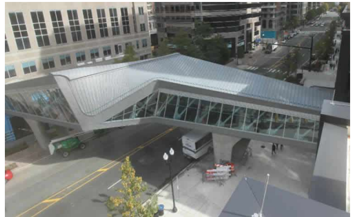
Exterior Picture of Ballston Quarter Pedestrian Walkway – Completed. Photo courtesy of ADTEK Engineers, Inc.
