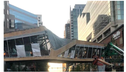
East Elevation of Ballston Quarter Pedestrian Walkway. Photo courtesy of ADTEK Engineers, Inc.
