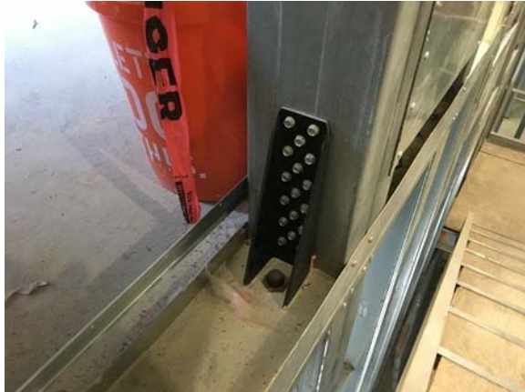
Interior hold-down with gypcrete – Photo by ClarkDietrich Engineering Services
