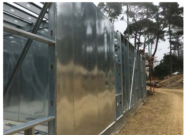
Exterior shear wall – Photo by ClarkDietrich Engineering Services
