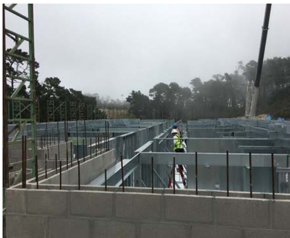
Top of walls – Photo by ClarkDietrich Engineering Services
