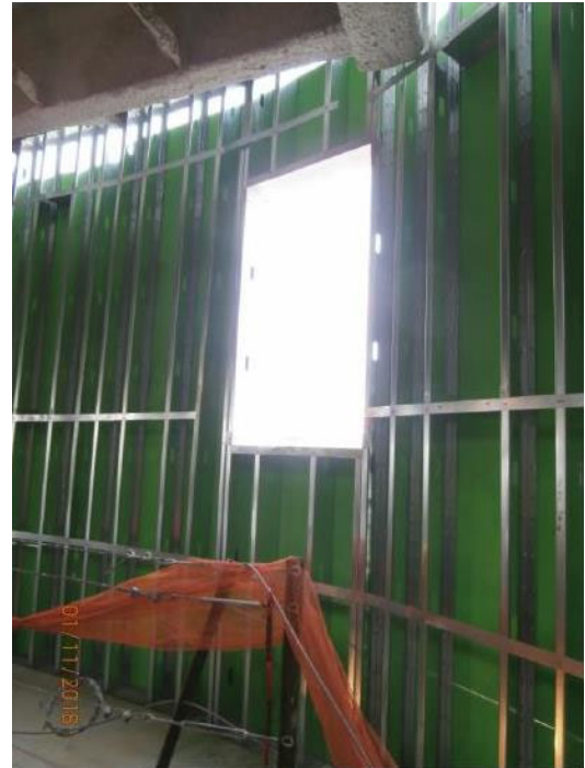
Interior image at curved punched opening to support eccentric window system
