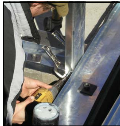
Electric screw gun with automatic feed nosepiece using bugle-head screws for sheathing attachment to steel.
