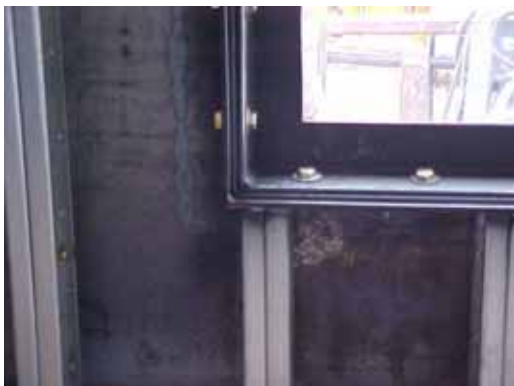
Figure 3: Typical window in test wall.
