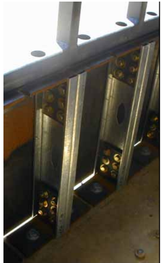
Figure 4: Upper floor window connection.
